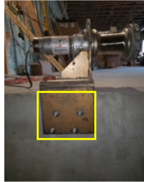
Figure 5 – Anchors installed on a shear
