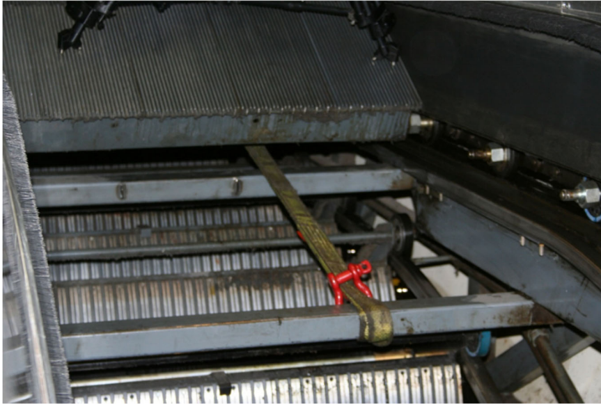
Step axles secured to the truss brace.
