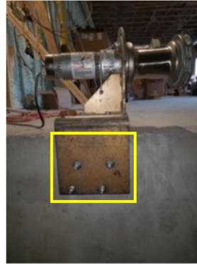
Figure 5 – Anchors installed on a shear
